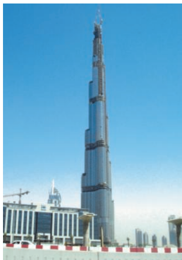
Dubai - Burj Khalifa - World's tallest tower under construction
